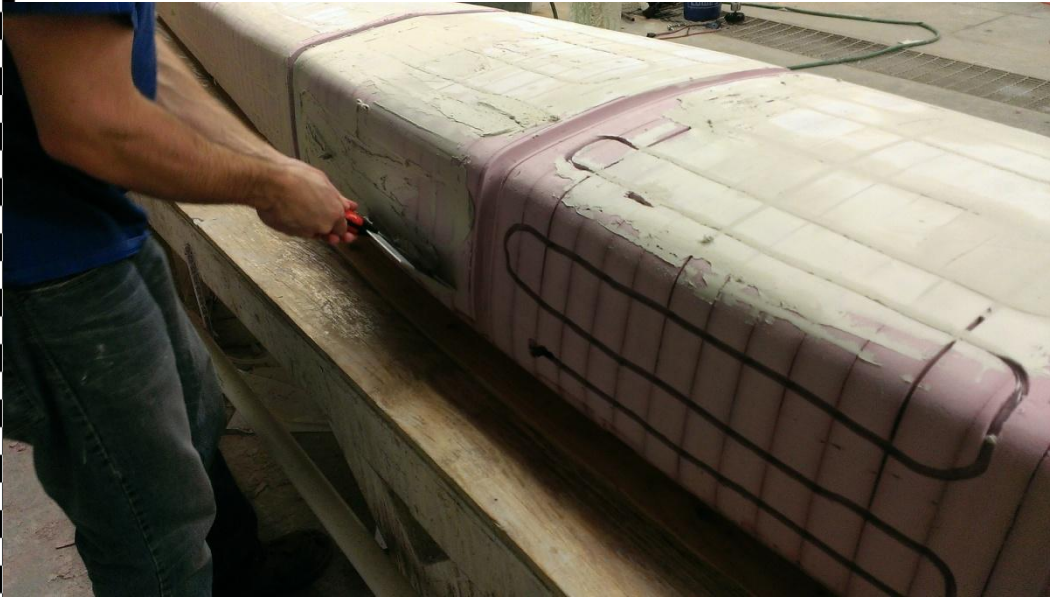
Covering the mold in drywall.
