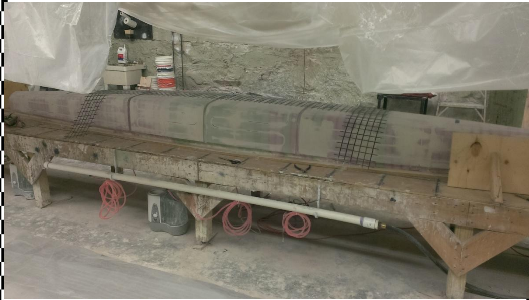
Mold fully assembled and prepped for placement day.
