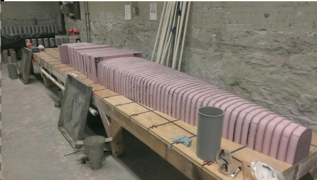
Cut foam sections laid out on placement table.
