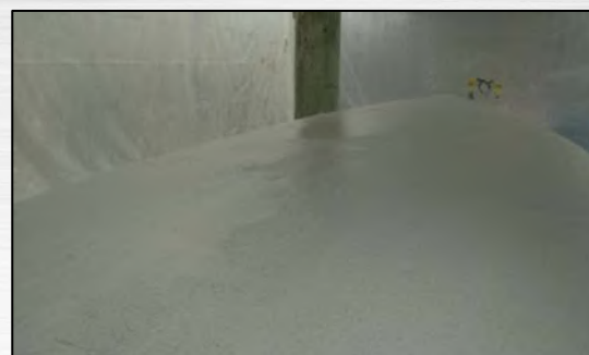
Figure 14. Trowel Finish of Backfire
